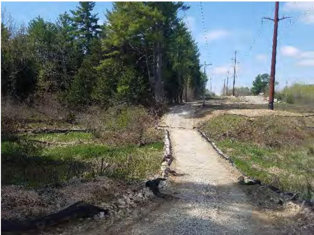
Fig 8: Access road between Strs. 51-52, over stream DS46. Viewing west. (05-15-20).
