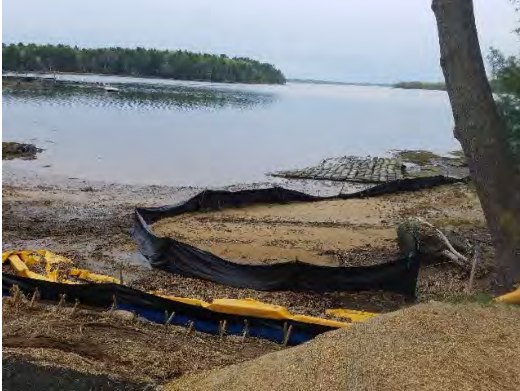
Fig 9: Settling of material for salt marsh restoration at Gundalow landing/east side of the Bay. Viewing west. (05-18-20).
