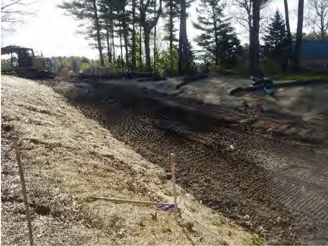
Fig 1: Rye Beach Landscaping spreading loam on slope at Gundalow landing/east side of the Bay. Viewing southeast. (05-14-20).
