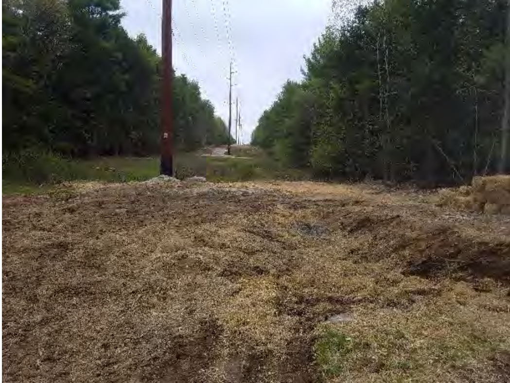
Fig 11: Str. 70 work area. Viewing east. (05-18-20).
