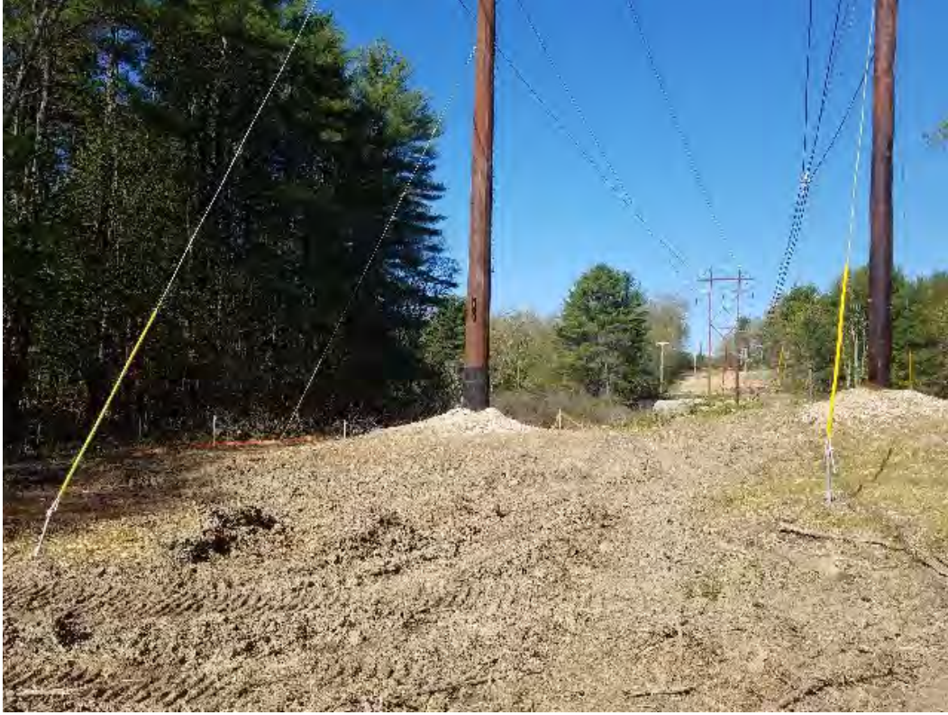
Fig 19: Str. 61 foundations. Viewing west. (05-20-20).
