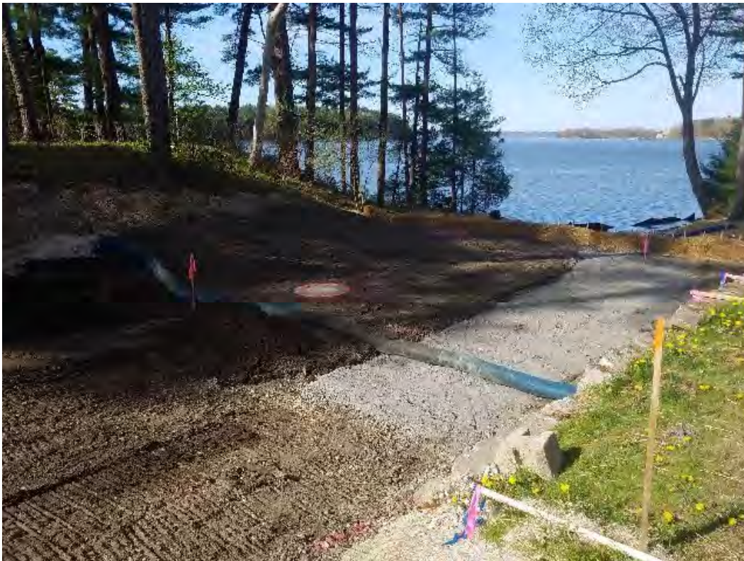
Fig 2: Rye Beach Landscaping spreading loam on slope at Gundalow landing/east side of the Bay. Viewing southwest. (05-14-20).
