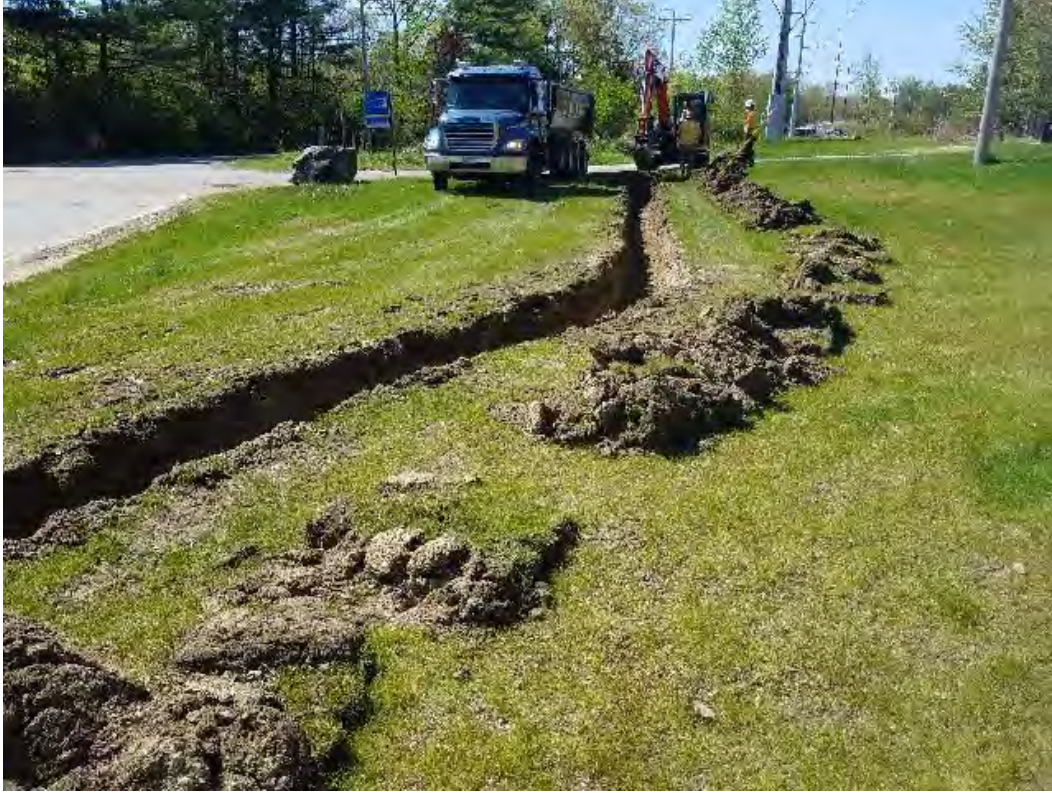
Fig 17: McCourt beginning to excavate for drainage repairs at UNH. Viewing south. (05-19-20).
