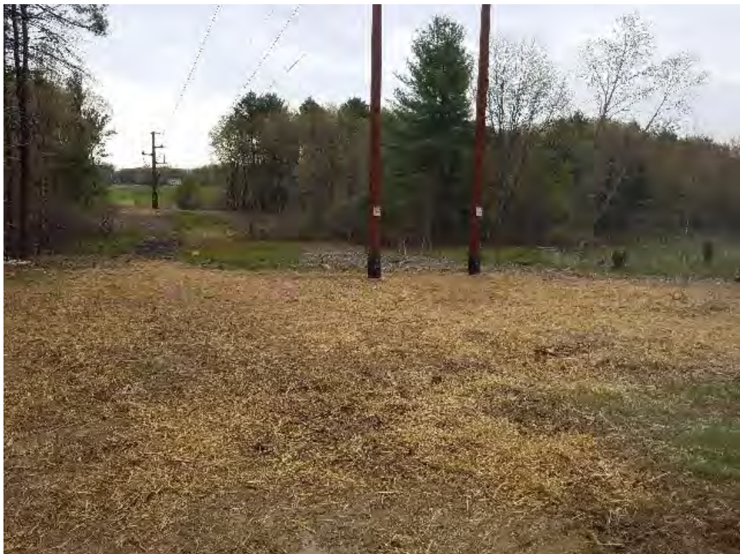
Fig 6: Str. 105 foundation and work area. Viewing northeast. (05-15-20).
