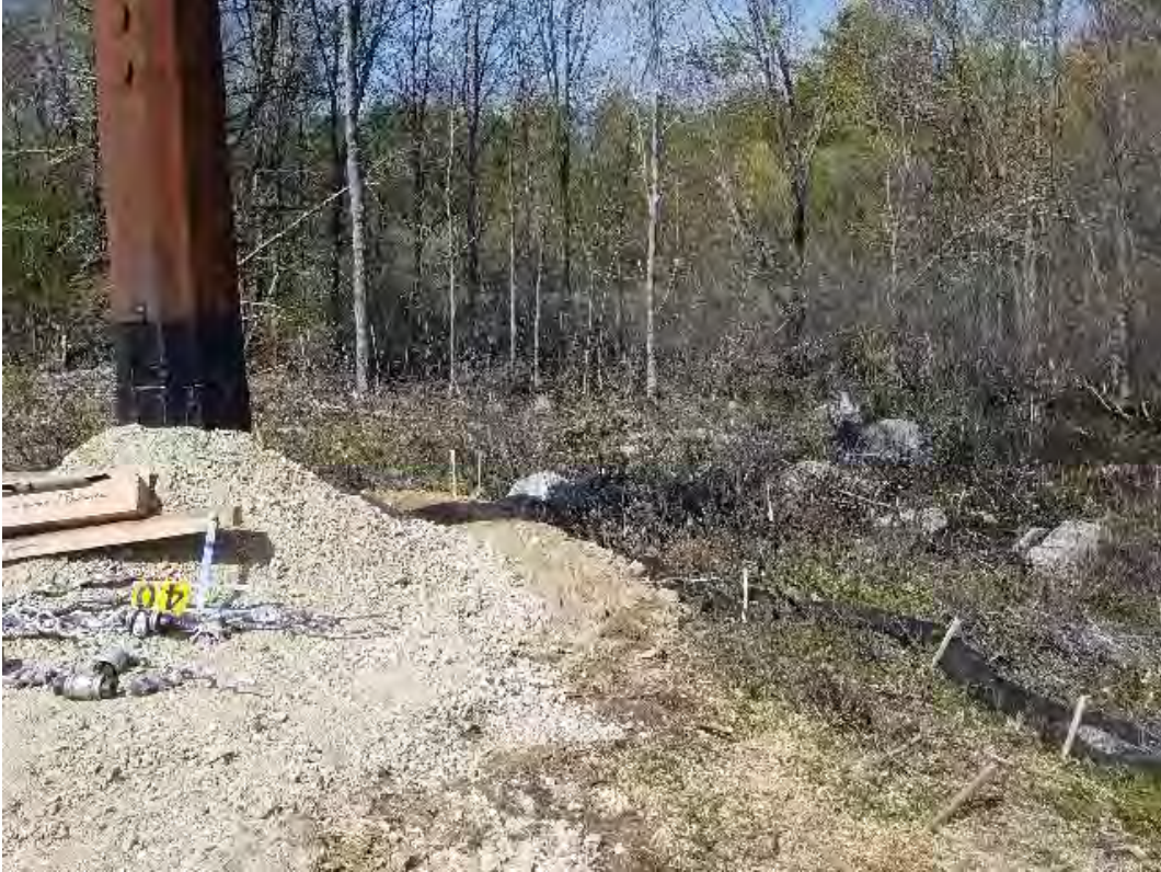
Fig 7: Str. 40 foundation. Viewing west. (05-15-20).
