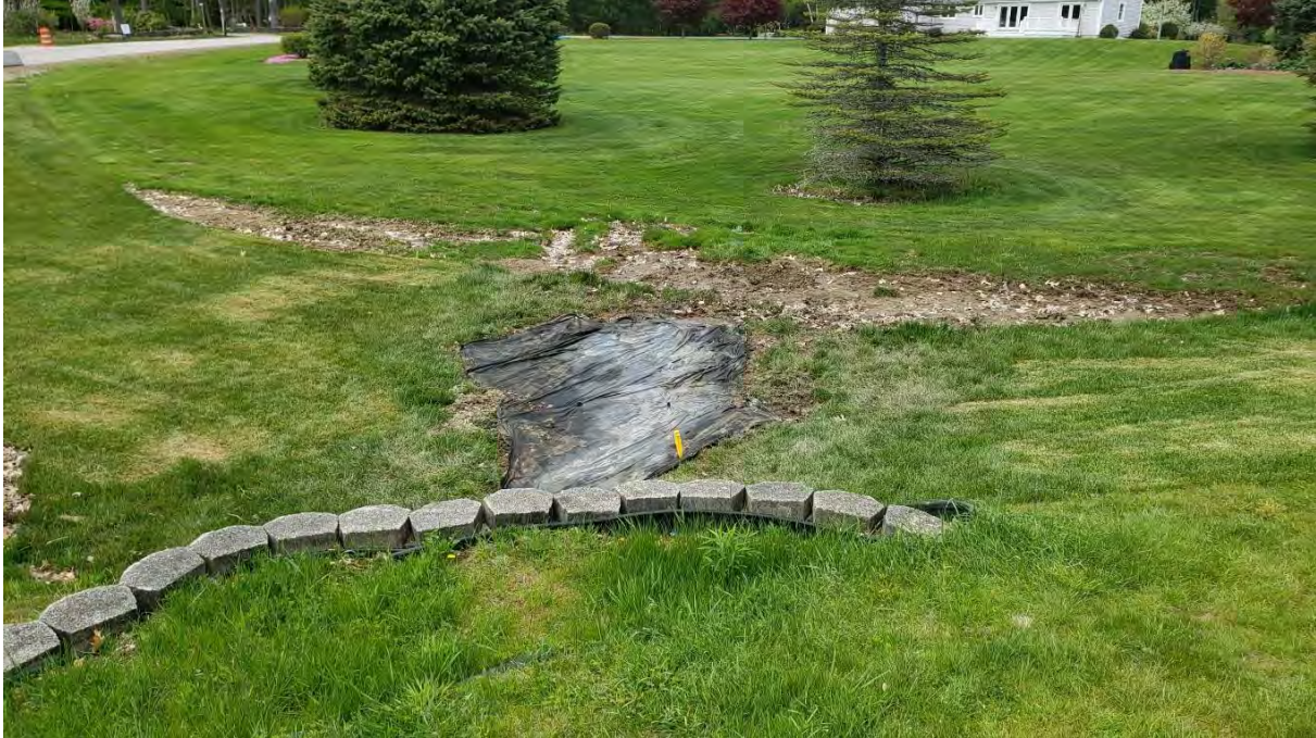
Fig 21: Seepage area on Veitas property. Viewing north. (05-20-20).
